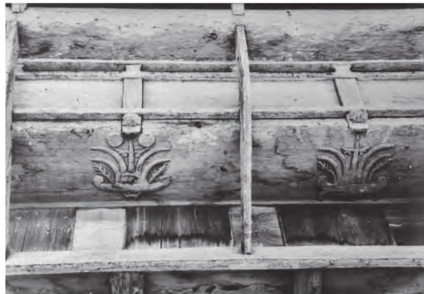
Fig. 7: Façade showing unpainted parts
