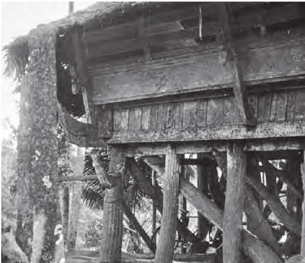
Fig. 10: Lasara on a central Nias chief's house between Orahili Village on the Eho River and the Susuwa River (Schröder 1917: Plate LXVI, Figure 127)
