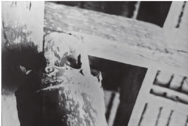
Fig. 13: Front pillar khölokhölo in the front room
