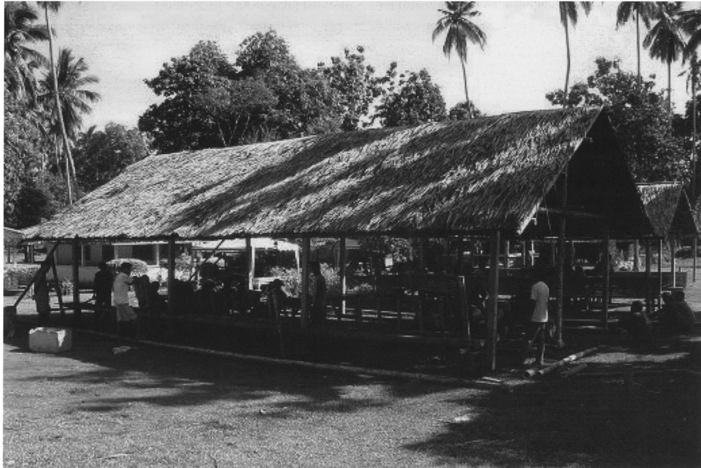
Figure 3. Hut under construction by coffee farmers, 2004 (photo taken by the author)
