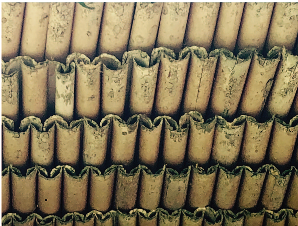
Figure 8. Simuane tallang roof detail. © Photograph: Aurora Donzelli.
