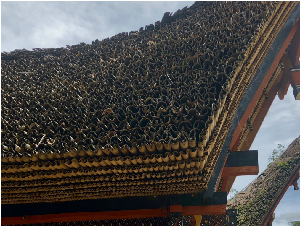
Figure 7. Bamboo roof illustrating the simuane tallang technique. © Photograph: Aurora Donzelli.
